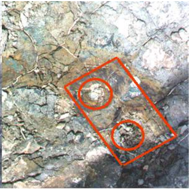
Illustration of the location of the plate and rivets. Notice the rust stains.
